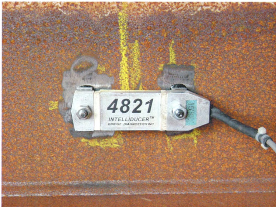
Figure 14. Details of gauge installation for various girder materials.
